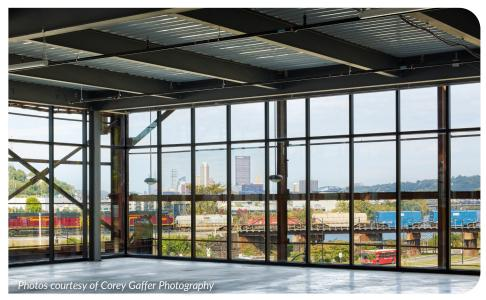
*Solarban*<sup>®</sup> 60 glass windows and *Solarban*<sup>®</sup> 70 glass skylights provide transparency and daylighting within the interstitial space between the historical steel cladding and new tech buildings.
